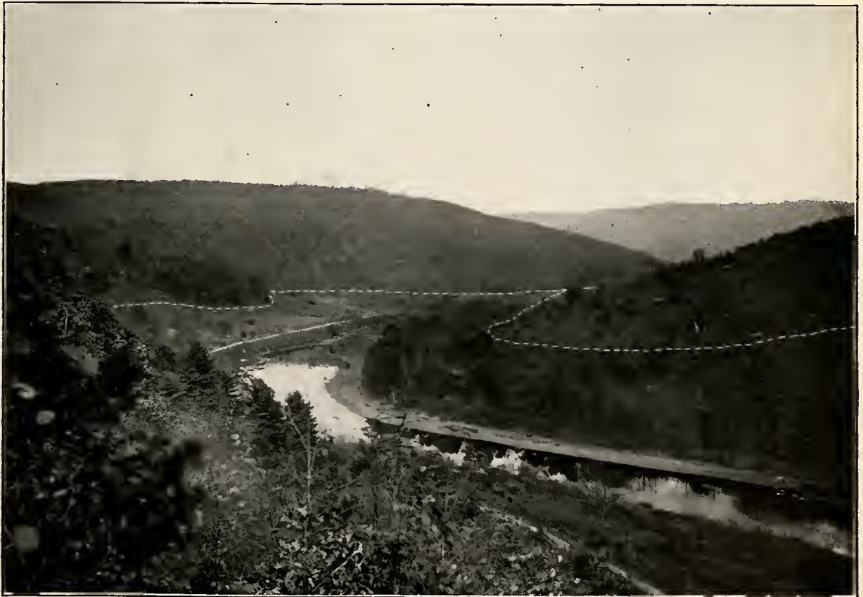
CLARION RIVER, PA., OCTOBER, 1910. View up stream, from a point 2.1 miles above Clarington; flow line of proposed reservoir No. 4 shown with dash line.
